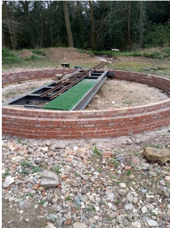
The new turntable nearing completion
