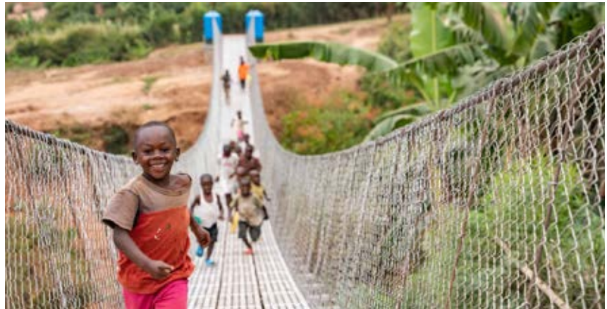
Enjoying crossing the new safe bridge at Nyacyonga – a gateway to opportunities.
